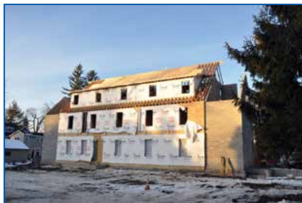
Stair towers at the rear corners of the house were installed, complete with steel stairs. This will be a fire-resistant escape route for all four levels of the facility.
