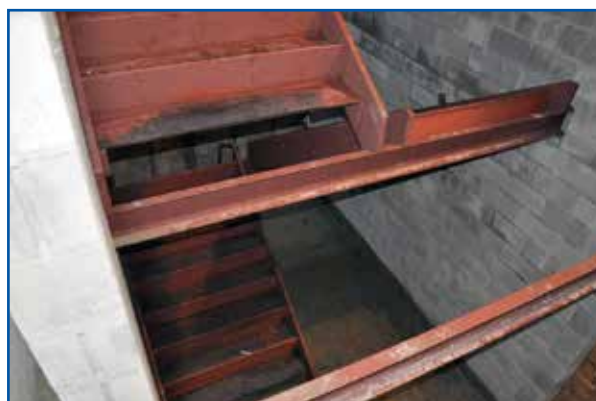
Stair towers at the rear corners of the house were installed, complete with steel stairs. This will be a fire-resistant escape route for all four levels of the facility.
